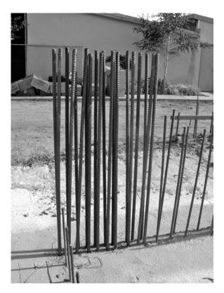
**Figure 10-17** Close placement of concrete shear wall jamb reinforcement calls for careful consolidation measures.
