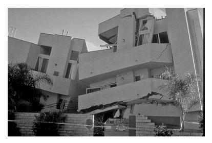
**Figure 8-6** Damage to building sustained in the Northridge Earthquake, California 1994. (*Courtesy UCLA Department of Earth and Space Sciences*)
