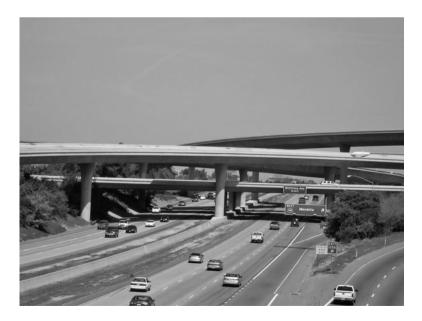
I Figure 5-4 Simple concrete grade-crossing bridges.
