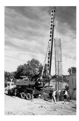
Figure 9-10 Placement of reinforcing bar cage into a drilled pier excavation. (Courtesy Conlan Engineering and Construction Corporation)
