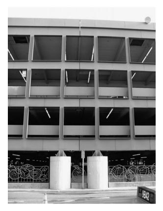
I Figure 8-17 Vierendeel truss configuration.
