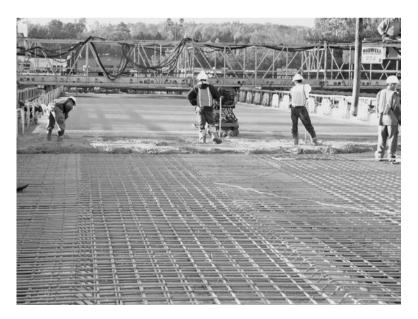
**Figure 5-5** Placement of concrete bridge deck. (Reproduced by permission of the Virginia Department of Transportation)
