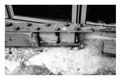
**Figure 7-6** Wood truss bottom chord tension failure. (*Courtesy Lane Engineers, Inc.*)
