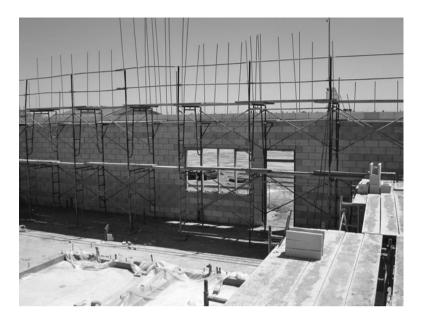
I Figure 11-1 Concrete masonry unit wall construction.
