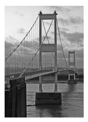
**Figure 5-6** Original Severn Bridge crossing between Wales and England, using a steel battledeck floor.
