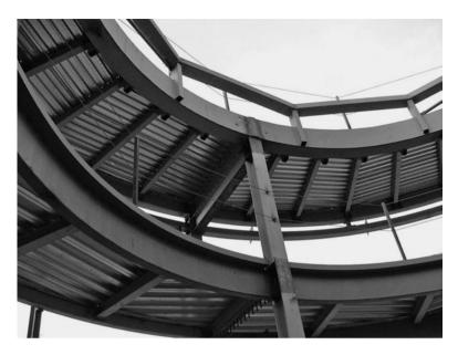
Figure 12-16 Rolled steel framing elements for roof and skylight system.
