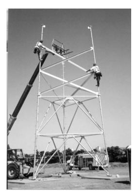
**Figure 7-4** Erection of structural steel-framed, antenna-supporting tower. (*Courtesy Conlan Engineering and Construction*)
