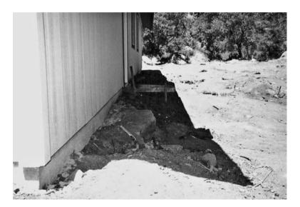
**Figure 9-5** Example of a poorly graded project site with standing boulders and loose soil.
