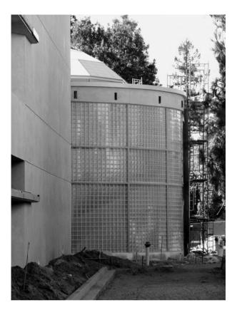
**Figure 11-5** Glass masonry walls provide beauty with structural strength, provided they are properly anchored to supporting elements.
