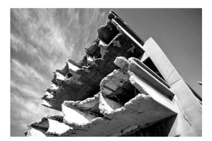
Figure 10-12 Concrete bridge damage from the Loma Prieta earthquake, California 1989.
