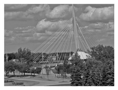
**Figure 5-9** Cable-stayed pedestrian bridge with added support for fabric shade canopy.
