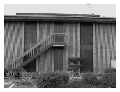
**Figure 4-5** Means of egress (exterior stairway) from second floor of a commercial building, which requires positive anchorage against a high live load under emergency conditions.
