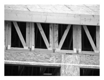
Figure 13-12 Anchored truss blocking panels to complete load path from diaphragm to shear wall.
