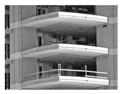
Figure 10-16 Concrete cantilevered slab elements may be designed as special plates using charts or simple computer analysis methods.
