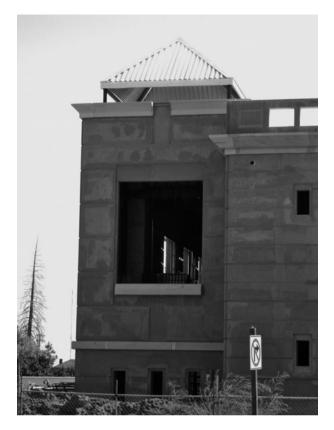
I Figure 6-2 Concrete shear wall system with openings.
