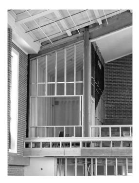
**Figure 3-5** Indoor mullion and steel framing with block out for glass panel, requiring consideration of solid anchorage against seismic shaking.
