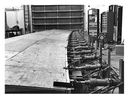
Figure 13-8 Horizontal plywood diaphragm testing. (Courtesy APA—The Engineered Wood Association)
