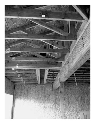
**Figure 13-17** Wood-frame trusses attached to structural beam, requiring hangers and consideration of shear wall placement for diaphragm shear transfer.
