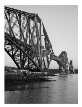
**Figure 5-3** Scotland's Forth Bridge, cantilever steel-type for railroad use.
