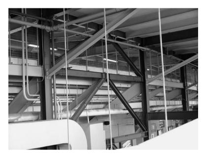
I Figure 8-16 Steel concentrically braced frame.
