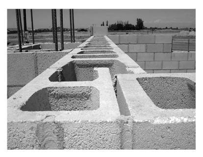
**Figure 11-8** Masonry walls may be constructed using blocks of differing widths for structural or architectural purposes.
