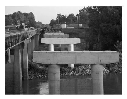
**Figure 5-15** Concrete piers for support of new bridge adjacent to existing bridge. (*Reproduced by permission of the Virginia Department of Transportation*)
