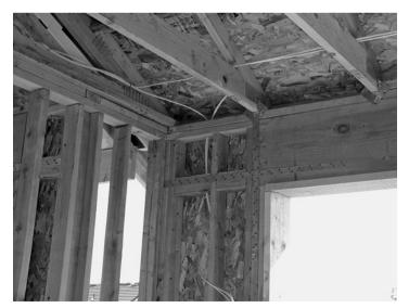
Figure 13-3 Steel straps installed at wood header to jack stud and horizontal blocking in narrow shear wall.
