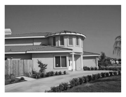
Figure 4-7 Roof diaphragms placed at different levels can present a challenge in tracing lateral forces to the foundation.
