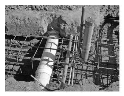
**Figure 9-9** Continuous footing with multiple pipes that may call for additional steel reinforcement.
