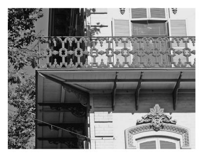
**Figure 3-6** Architectural railing system in need of structural anchorage against code-required horizontal forces, New Orleans.
