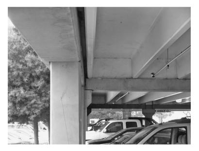
**Figure 10-8** Bearing conditions of precast concrete sections in a parking garage.
