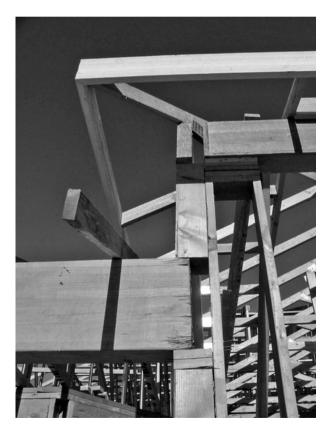
**Figure 4-11** Poor wood-frame construction detail with lack of proper load path and connections.
